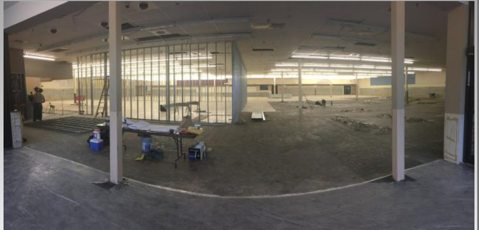
January 13, 2020 – Framing begins on interior walls.
