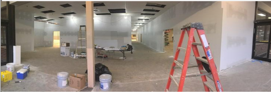
February 20, 2020 – Walls are completed and prepped for painting.
